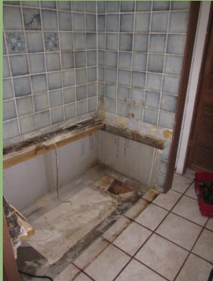
Preparing a tub/shower install
